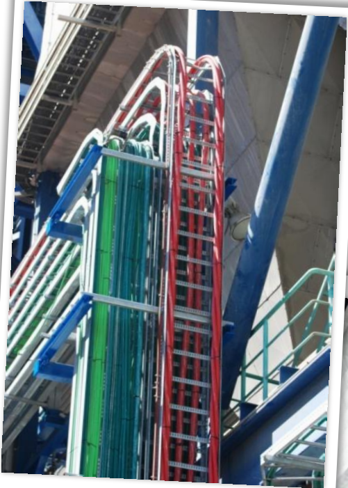
Litoral Power Plant (ENEL) Carboneras (Spagna)
