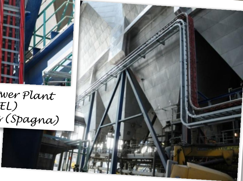
Litoral Power Plant (ENEL) Carboneras (Spagna)
